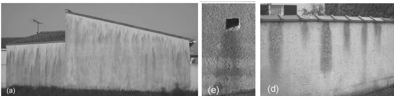
Figure 6. Images of the locations in France of collected samples, showing the different levels of bio-growth on a wall surface depending on the conditions of water content. From left to right: a) on mortar located along the Atlantic coast, extensive red colonisation by *Trentepohlia iolithus* was found, d & e) from zones of high micro-humidity black stains were collected composed of algae and cyanobacteria.
