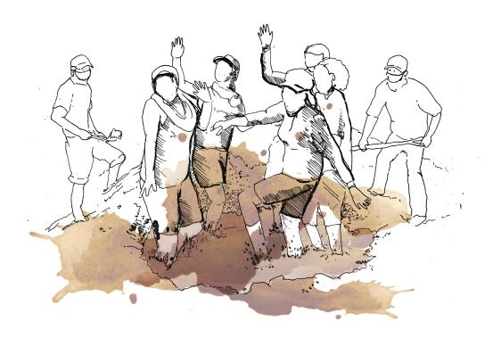
A simple recipe of earth, water and sand. The mixture can be prepared by all ages. Like kneading dough, the mixture of la quincha can be adjusted to suit the required outcome. The action takes place on the ground, a pit to be precise. There is no precision to the quantities of material, however. The experimental notion of the act, gives an authenticity to the Valparaisan way of life.
