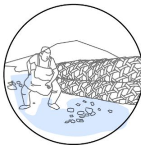
Rebuild Bamboo Cage Weir
