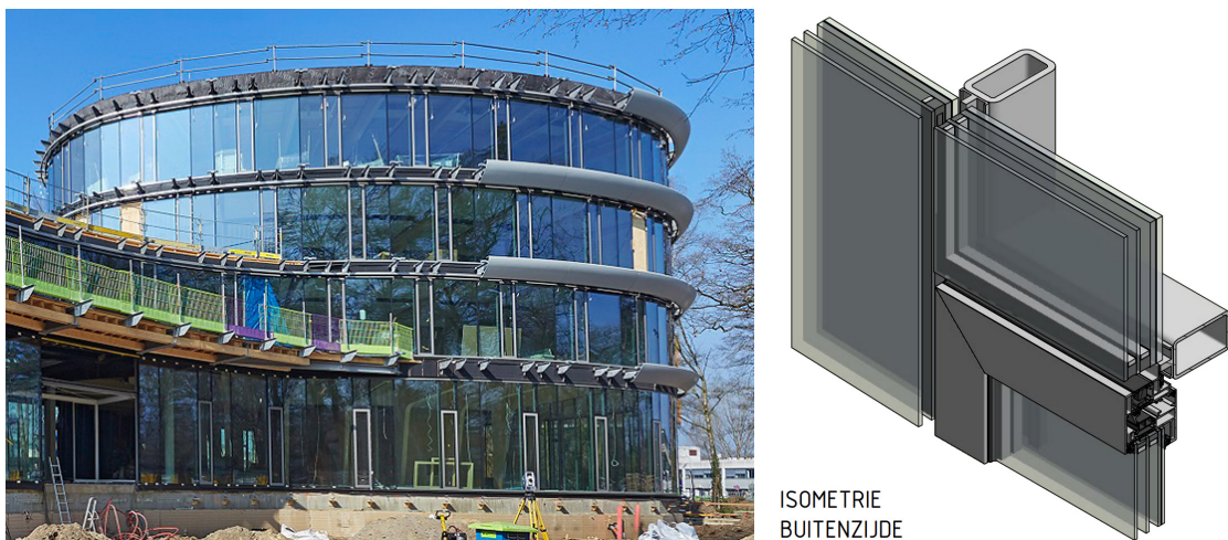
Figure 3.57. (left) Triodos Bank Façade in Driebergen-Rijsenburg, Netherlands. (right) Typical Façade Detail of Triodos Bank analyzed in this research. Adapted from (Octatube, 2018).
