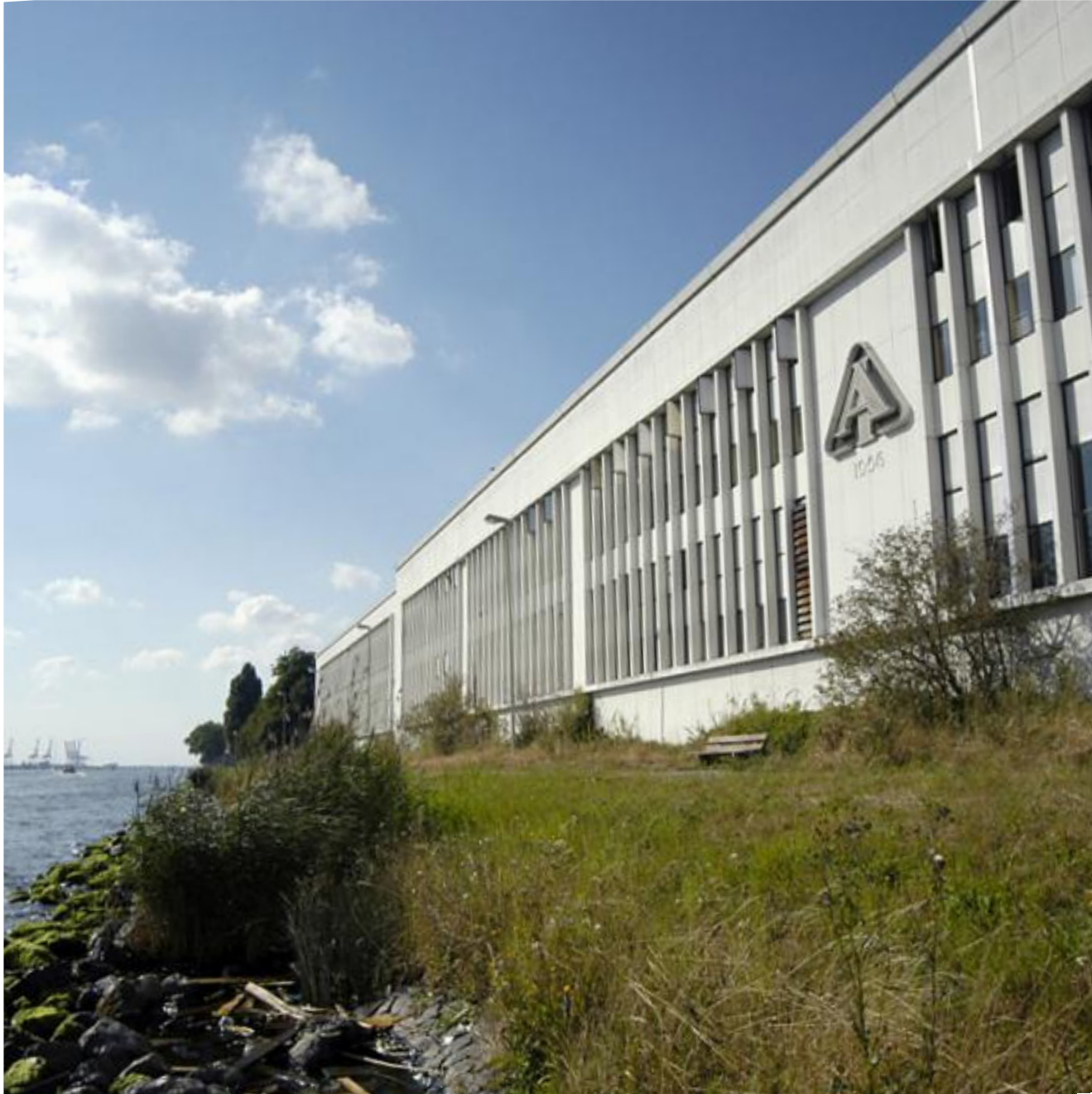
View of Building 429, along Hemkade. © nul20.nl
