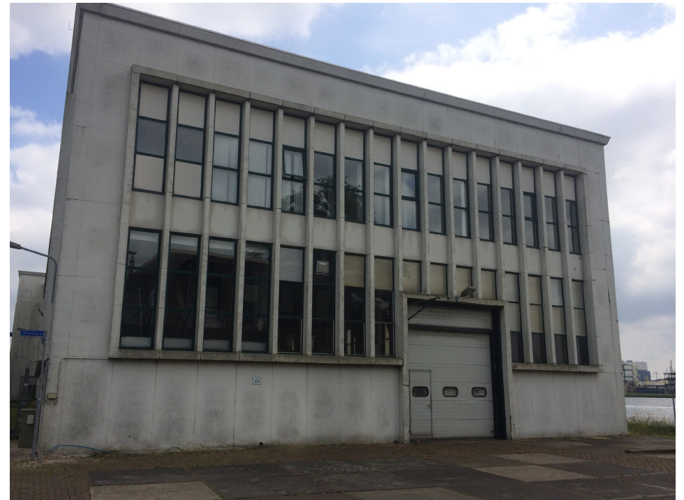
View of Building 429. © Bill Iliopoulos
