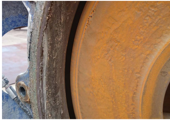
Figure 3.13: Suction Shroud after pumping 33.000 TDS
