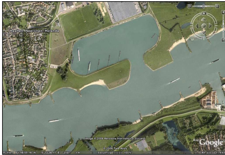
Figure 1.1. Port of Haften, River Waal. The Netherlands.
