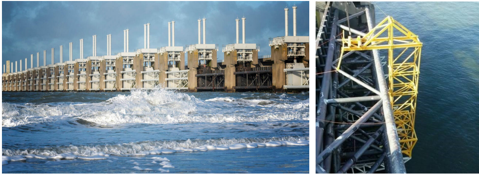
Figure 1.2: The Eastern Scheldt barrier in the Netherlands (ref: Rijkswaterstaat). Wave impacts have played a major role in the design of the gates. Also the recently implemented temporary maintenance structure at the backside of the gates can be subjected to wave impacts.
