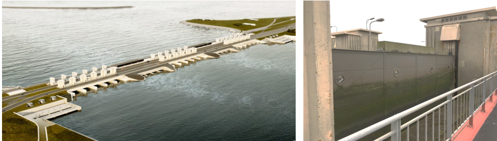
Figure 1.3: The design for the Afsluitdijk renovation (ref: Level) and one of the gates in the existing discharge sluices. Both the existing and newly designed gates may be subjected to confined wave impacts due to overhanging elements.
