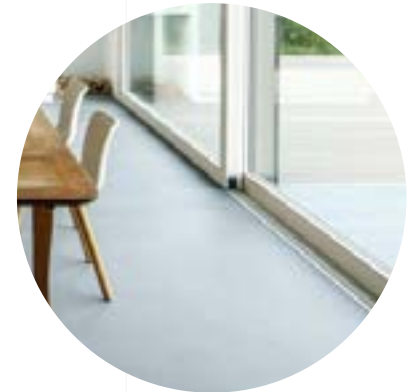
POLISHED CONCRETE FLOOR IN CIRUCULATION AREAS
