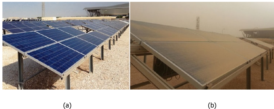
Figure 1.7: Module soiling due to the sandstorm event observed in Qatar, Doha [38].
