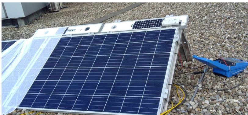
Figure 2.16: Placing of white fabric to simulate uniform soiling of 30% T_{loss} .
