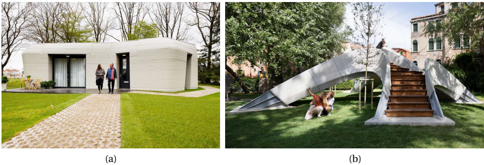
Figure 2.3: Case studies 3DCP a) Milestone house [42] b) The Striatum bridge [43]
