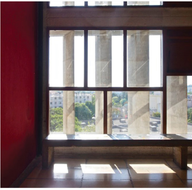
Brise soleil Source: Radiant City: The Marseilles Housing Unit (2017) Retrived at: https://bit.ly/2laho3Q
