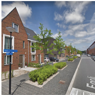
Renovation projects in Biljmermeer Source: Failed architecture https://goo.gl/XMS5N
