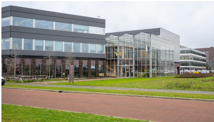
Figure 4.2: Biopartner after construction (LBSPG, n.d.)
