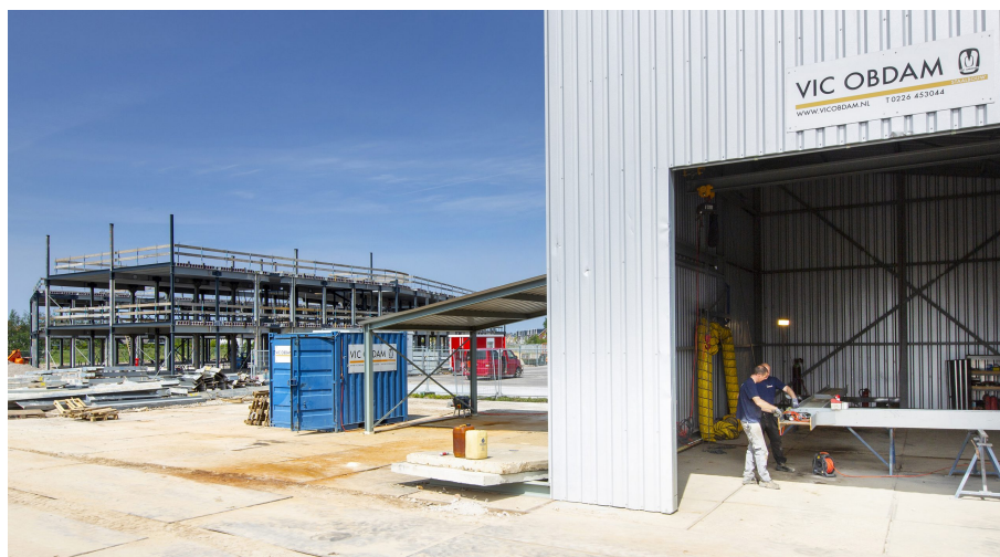
Figure 4.7: On-site workplace for steelwork by Vic Obdam (Beenker, 2021)
