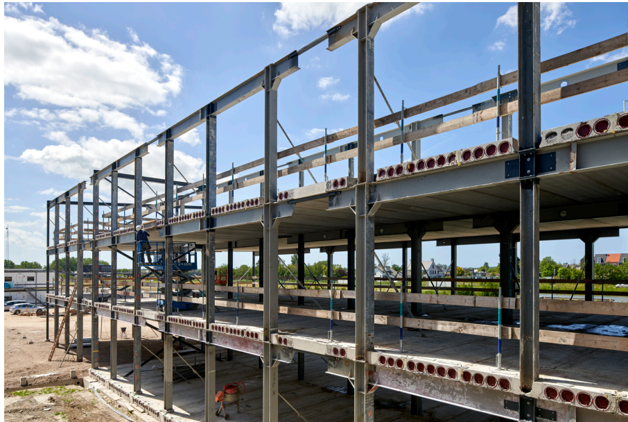
Figure 4.4: Reclaimed steel portals used in the Biopartner 5 steel frame (Beenker, 2021)
