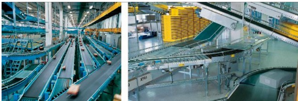
Figure 2.2: Complicated conveyor belt system
