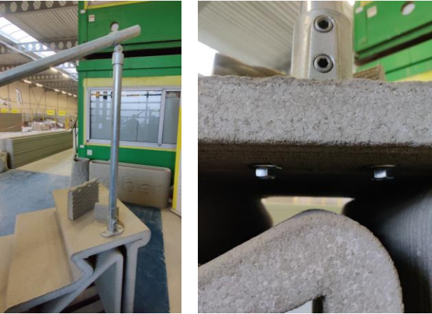
Figure 48: Steel handrail connected to 3D-printed structure with bolts
