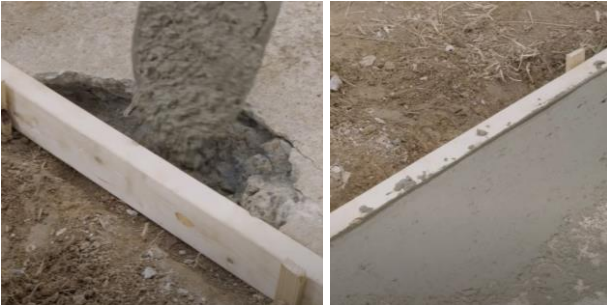
Figure 50: Repair with wooden form box [227]
