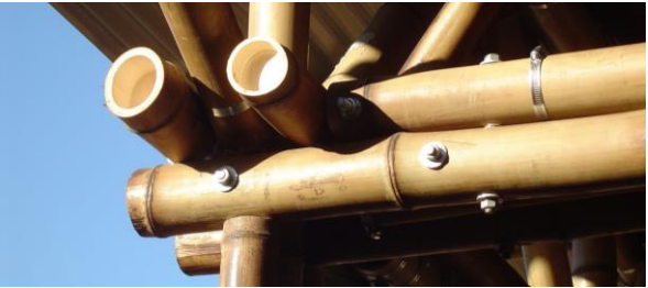
Figure 78: Bamboo bolt connection [285]
