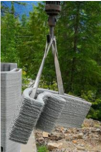
Figure 64: Lifting 3D-printed concrete stairs [275]
