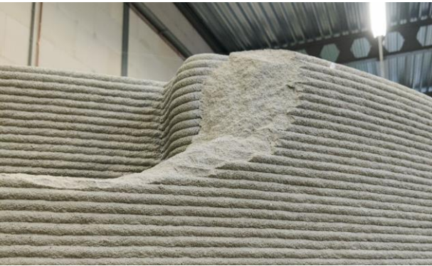
Figure 49: Damaged 3D-printed structure at Weber
