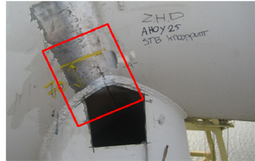
Figure 14: Past found cracks
