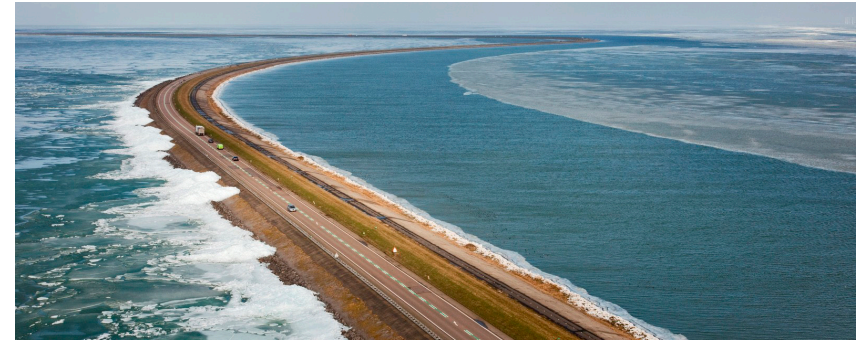
Grey infrastructure: Houtrib dike in the Netherlands Source: Van Oord
