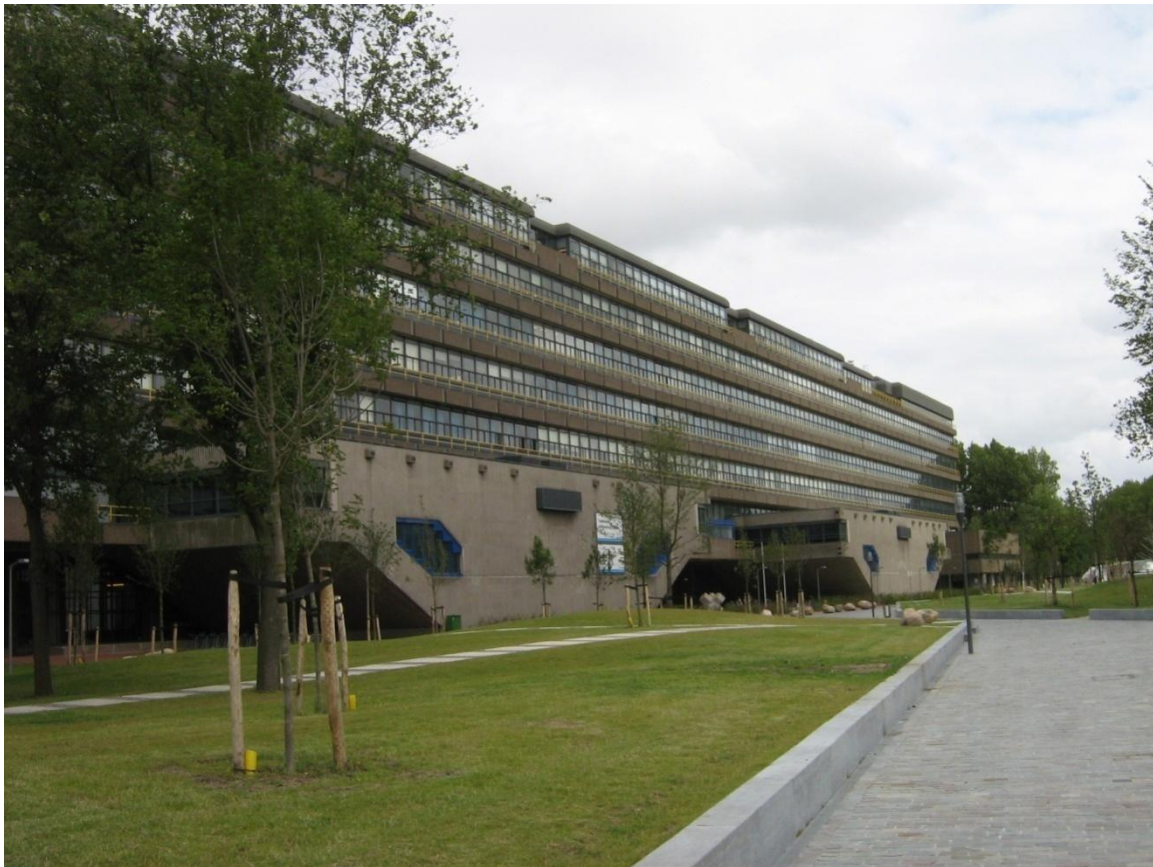
Figure 1.1 Faculty building of Civil engineering and Geosciences
