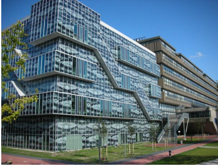
Figure 3.2 Refurbished façade of the faculty of geosciences (photo by T. Ebbert)
