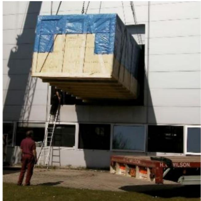
Figure 3.2: The delivery of SIMONA's collimating mirror. Image courtesy of ir. Olaf Stroosma.
