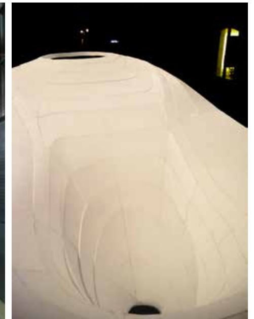
Leuven Pavillion. Technique: Robotically cut EPS modules.
