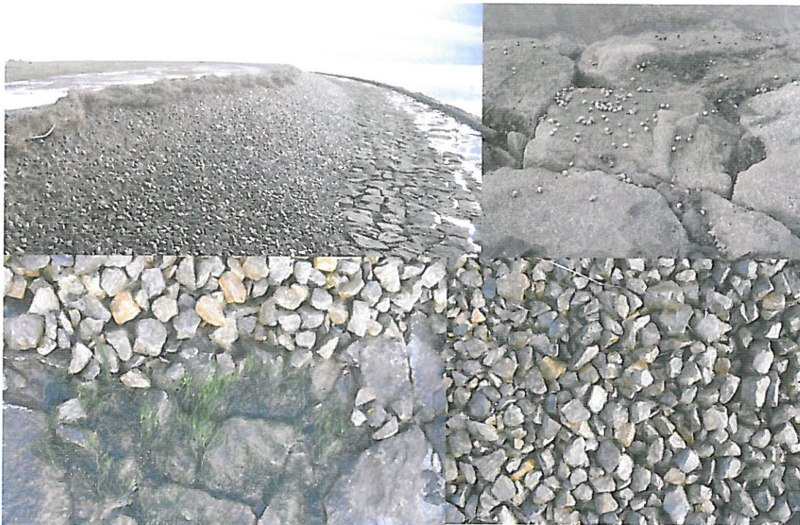
Figure 25. The top left part shows an overview of the second Hallig Gröde pilot. There is no vegetation on the Elastocoast layer (bottom right), but sometimes there is Blidingia minima on the basalt below (bottom left). The only animals found on HG2 are
