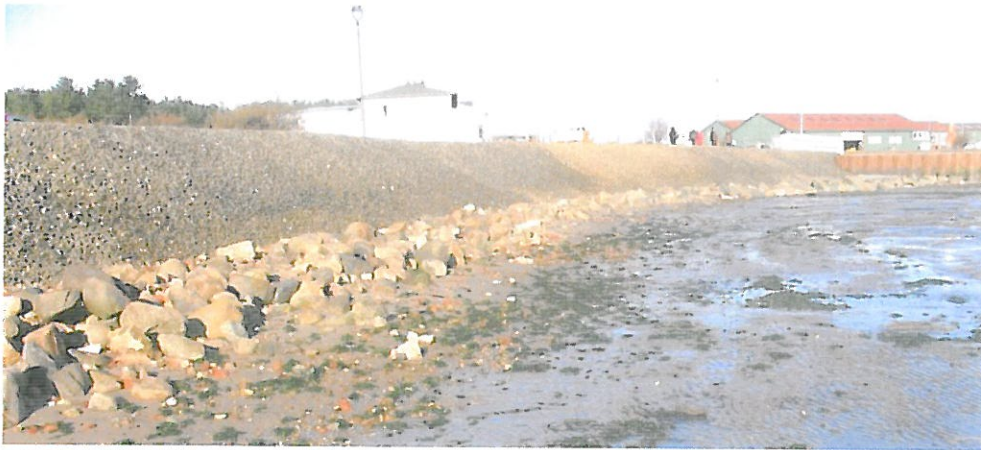
Figure 27. The Elastocoast revetment of Sylt Munckmarsch. Notice the algae on the sand. Although there are no algae yet on the revetment, the green algae from the sand might migrate upwards.
