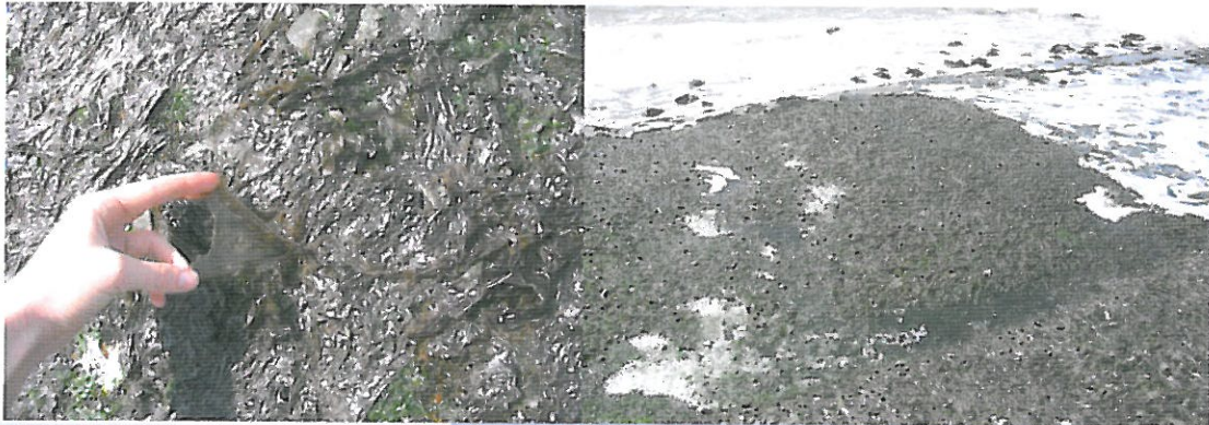
Figure 35. Top left: A Furoid algae. Top right: tidal pools filled with water at low tide. Bottom left: The Elastocoast layer is covered with algae. Bottom right: an overview of the Petten revetment. Note the birds on the layer.
