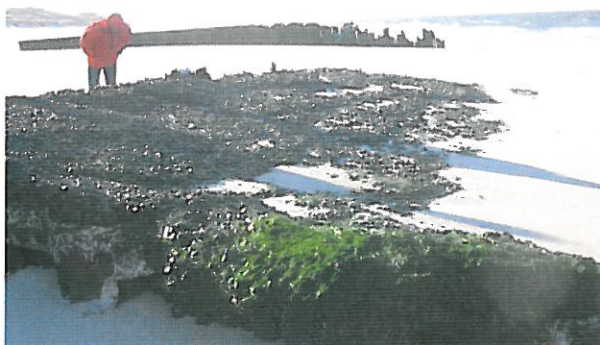
Figure 26. The Elastocoast site on Sylt Ellenbogen. On the parts of the shore, Blidingia minima is growing.
