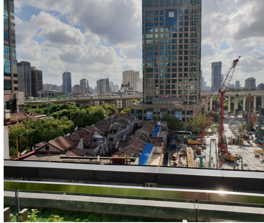
City redevelopment in the city of Shanghai in 2018. Here one form of spatial density, the lowrise neighbourhood, is removed to make place for a different typology, that of the commercial and/or residential tower. One could question what the effect on the use of public space will be.
