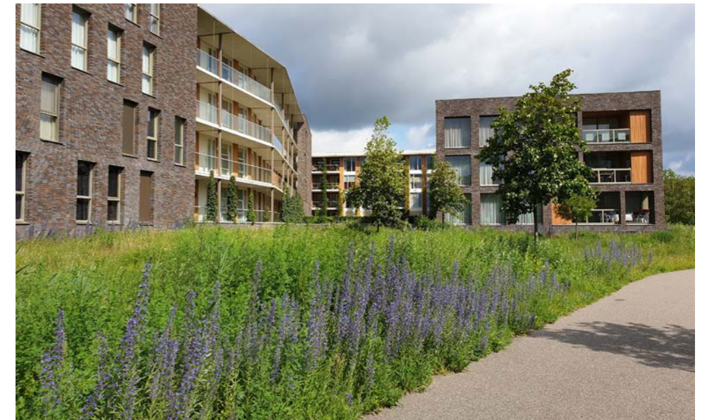
The park around Annenborch elder care building in Rosmalen, 's-Hertogenbosch, 2019. Here the green space not only provides support and regulatory ecosystem services, but it is an important part of the privacy zoning.
