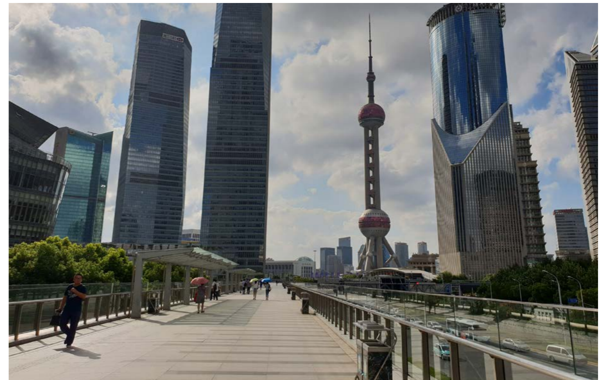
One of the elevated walkways at Pudong, Shanghai in 2018. Here the conflict between pedestrians automobiles has been used to create a totally new elevated infrastructure that functions as a place as it not only connects different buildings, but also allows for optional and social activities as part of the identity of the Pudong district.
