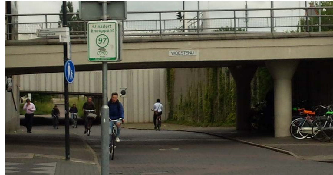
The aptly named tunnel/bridge Woestenij or Wasteland, near Eindhoven station in 2018. Conceived as a solution to the conflict between active mobility and the automobile near Eindhoven train station. Although the conflict has been resolved, the resulting spatial quality of the route discourages optional activities or social activities, resulting in a non-place.
