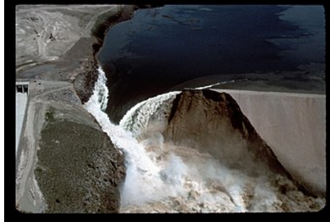
Figure 1.6: Teton Dam: Catastrophic failure on June 5, 1976 [59]
