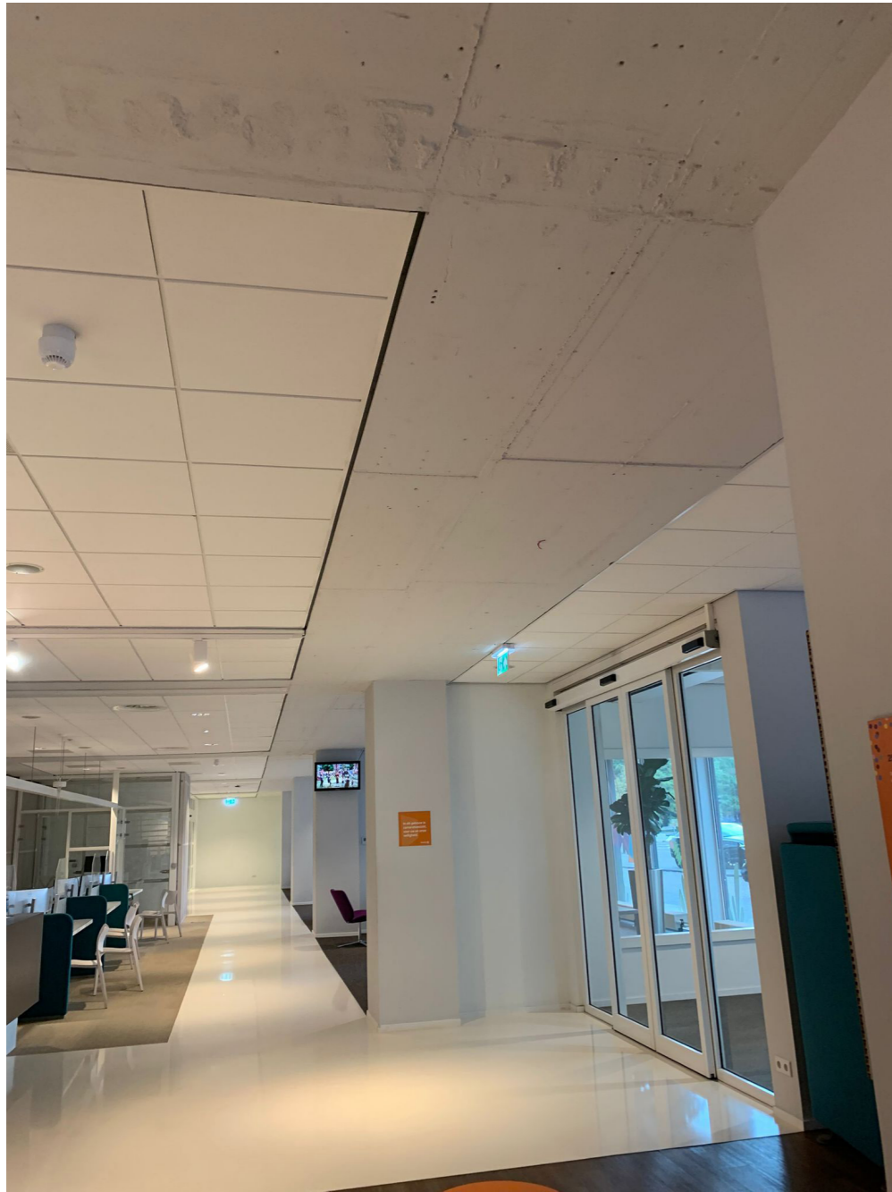
concrete beam - ground floor
