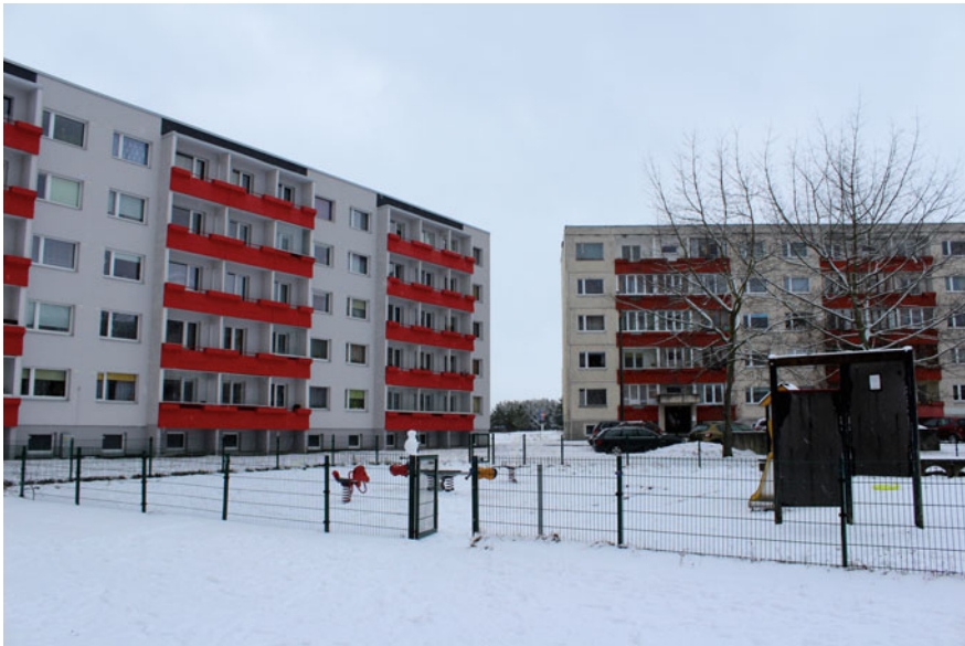
Fig. 17.6 Apartment building after undergoing KredEx-funded renovations on the left vs. an unrenovated apartment building on the right. Source Annika Väiko
