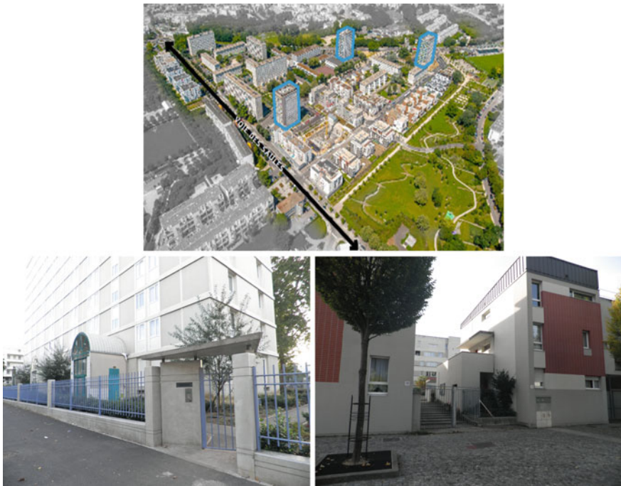
Fig. 14.6 ‘Gating’ of existing buildings and new housing developments in Orly
