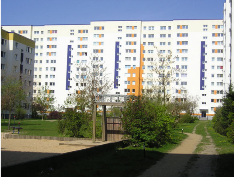
Fig. 5.7 A large courtyard in Marzahn built in the 1970s; renovated and fitted with insulation and colourful façades in the 1990s. Source Florian Urban, 2005
