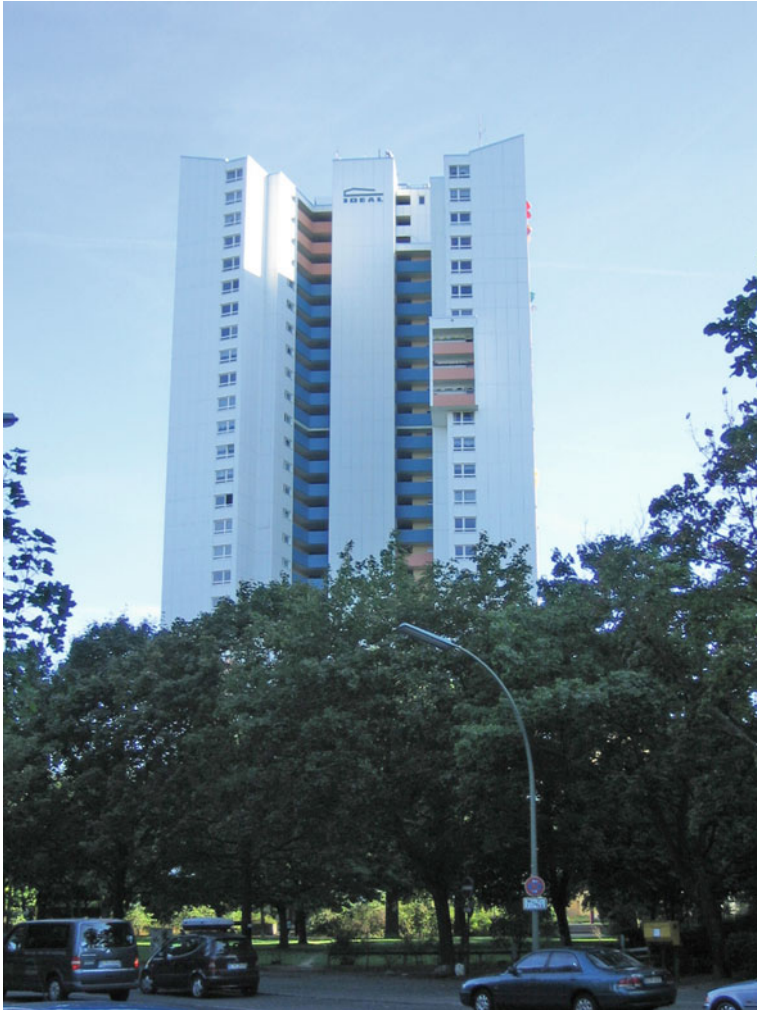
Fig. 5.5 The ‘Ideal Tower’ (1966–1969, Walter Gropius/Alexander Sviranovic), commissioned by the Ideal Construction Cooperative in the Gropiusstadt estate in West Berlin. Source Wikimedia Commons/Magnus Manske, 2008
