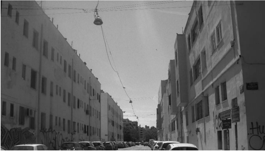
Fig. 4.1 The first four condominiums in Dourgouti, part of the old public housing stock for refugees constructed between 1935 and 1936 by the Ministry of Social Care, 2016. Source Myofa, personal archive, 2016
