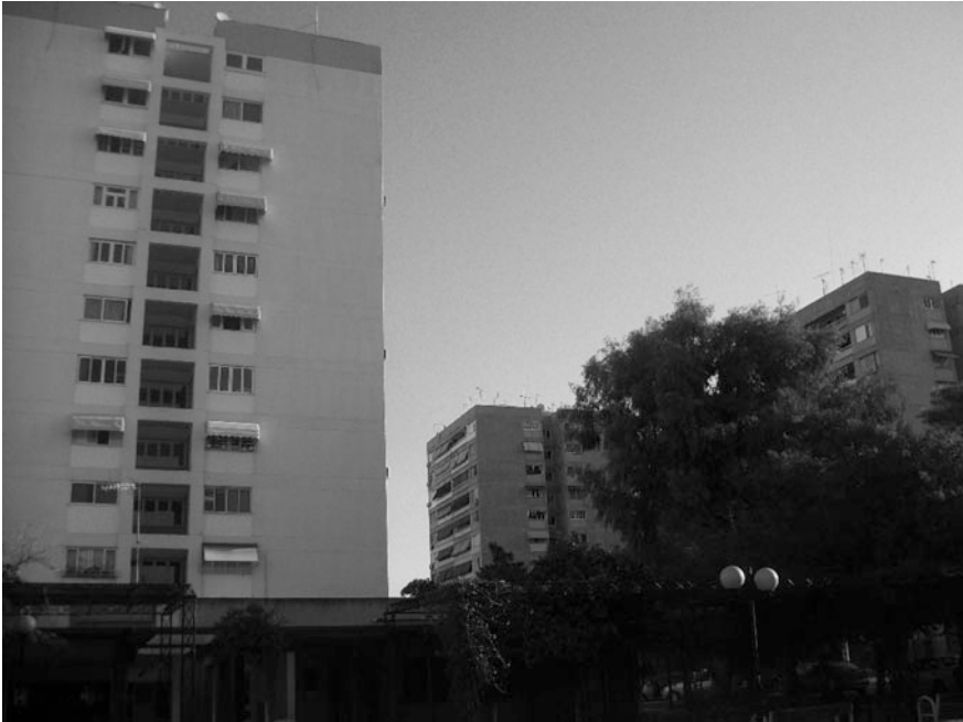
Fig. 4.4 Ten-storey condominiums in Tavros built between 1969 and 1971 by the Ministry of Social Care, 2016. Source Myofa, personal archive, 2016
