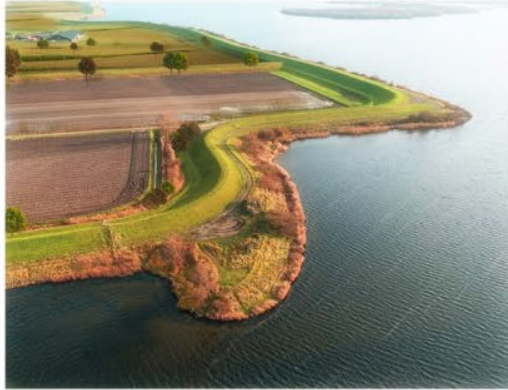
[Fig. 45] Existing situation
