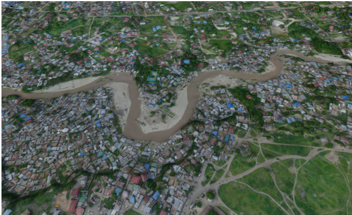
Figure 3.7: Build up sections of flood banks along the Jangwani Bridge. These build up regions can be found along the banks of all rivers in Dar es Salaam. (Ramani Huria, Dar Es Salaam, 2019)
