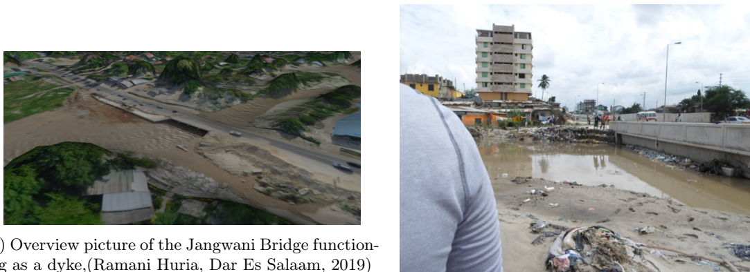
(b) The Jangwani bridge clearly functions as a dike in this picture.
