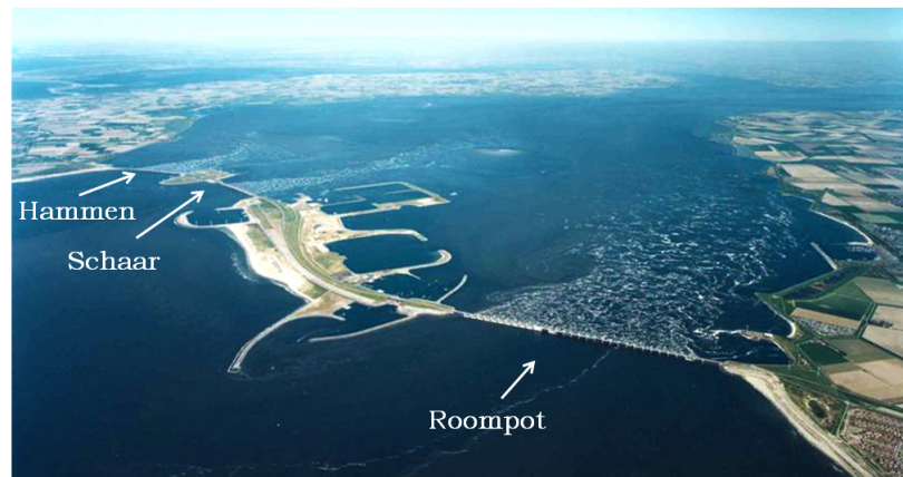
Figure 1.2: Aerial picture of Eastern Scheldt barrier, seen from the west (Biesboer, 2011)
