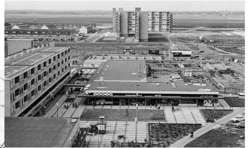
Hoge Vught in construction in 1971 (Source: Steenhoven, 2019)
