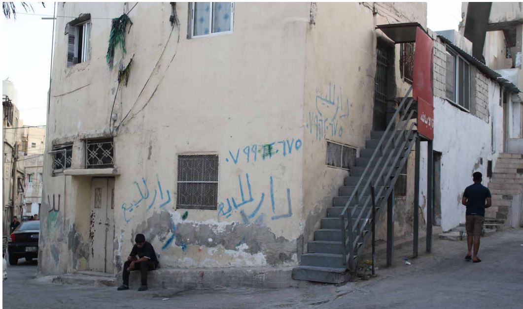
FIG. 6.7 External steel stairs connecting floors on the outside, extending beyond the parameter of the unit.
