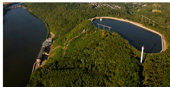
Figure 3.1.3: Example of a 152 MW pumped hydroelectric storage facility Koepchenwerk, Germany. Image reprinted from Entura (2016)
