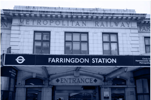
Fig.57 - Author's work, Farringdon station entrance
