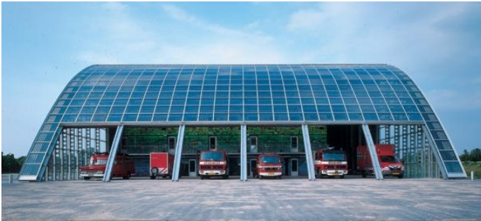
Figure 1.4: The fire station of Houten/Utrecht as an example for different module orientations as a consequence of building integration [51].
