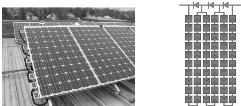
Figure 4.30: Left: The back row of the two monitored module strings (the front row is not visible in the picture). Six silicon sensors that measure the irradiance in 5-minute steps are installed along the left-hand edge of the back row modules. Source: QPV group of Fraunhofer ISE. Right: The circuit diagram of a standard c-Si PV module made of 60 PV cells (here: Sunways SM 215 WA63). All c-Si cells are connected in series; one bypass diode protects 20 PV cells.
