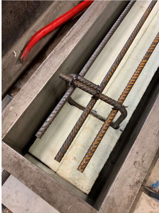
Figure 2-7: slots in the Styrofoam inside mould to place the stirrups in
