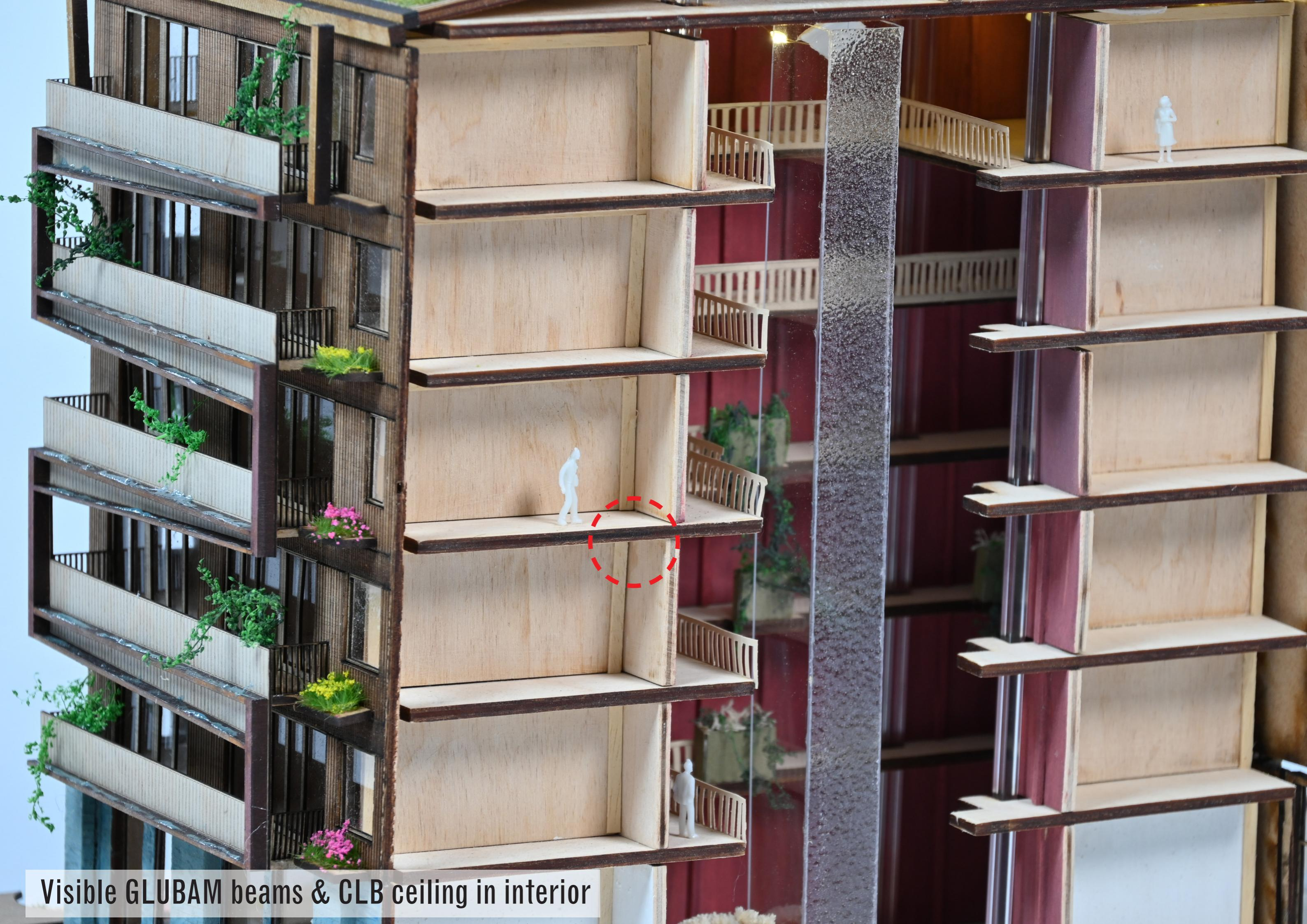
Visible GLUBAM beams & CLB ceiling in interior
