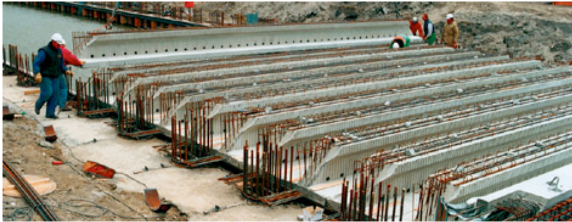
(a) Prefab inverted T-profiles put into place [68]
