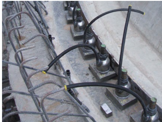
(b) Application of bonded post-tensioned bars [83]
