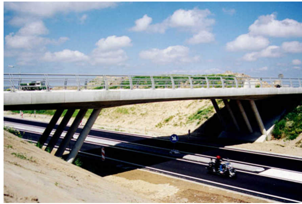
Figure 2.55: Example of a “springwerk” viaduct, characterised by its inclined piers [87]
