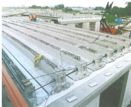
(a) Construction of girder bridge with transversal reinforcement for crossbeam at support put in place [65]
