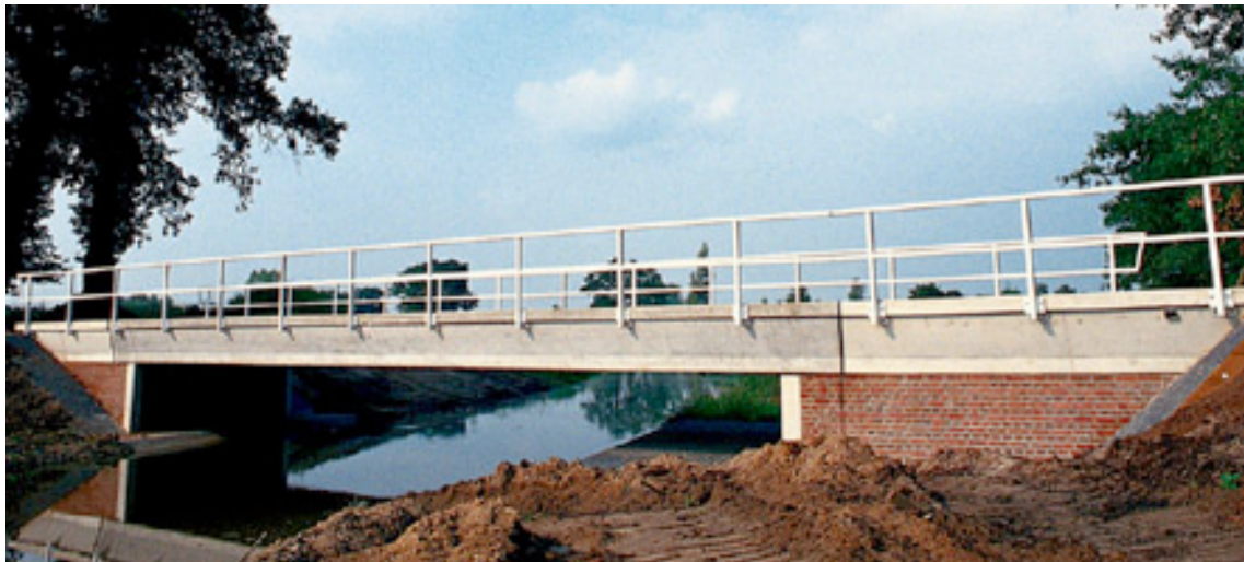
(b) Finished solid slab bridge [68]
