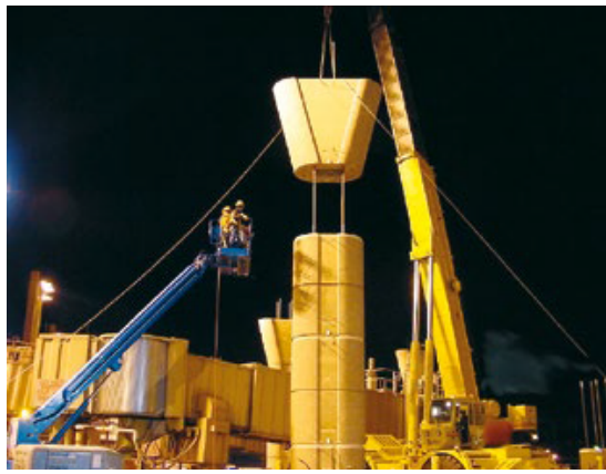
(a) Assembly of prefab elements into a pier [83]
