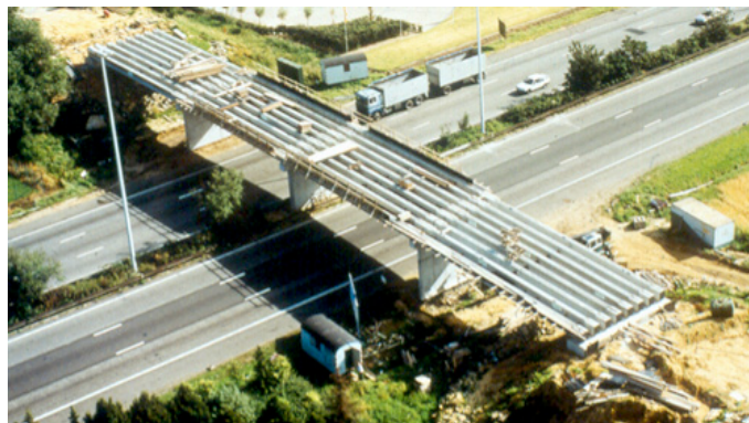
(b) Construction of girder bridge over highway with no traffic interruption [68]
