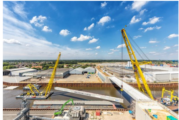
(b) Construction of Lienebrug in Wanssum (NL) with world record-length box beams of 69 m [77]
