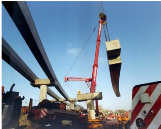
(a) Construction of box beam bridge for metro rail in Amsterdam [65]
