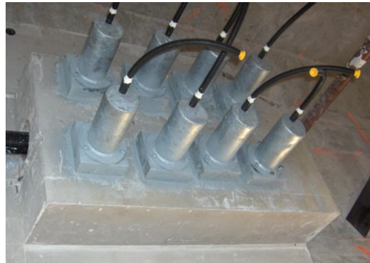
(b) Application of unbonded post-tensioned bars [83]
