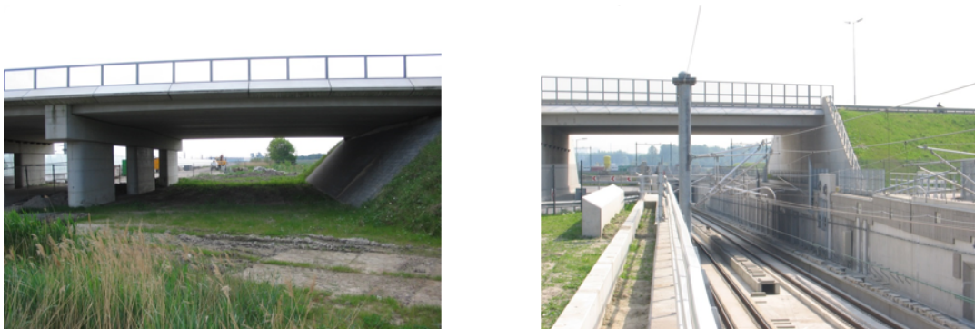
Figure 2.33: Examples of a viaduct with a bank seat (left) and a viaduct with an abutment, crossing a railway track (right) [65]
