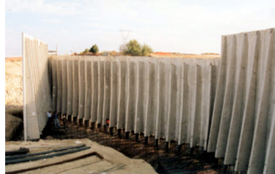
(b) Example of prefabricated abutment with ribbed wall [68]
