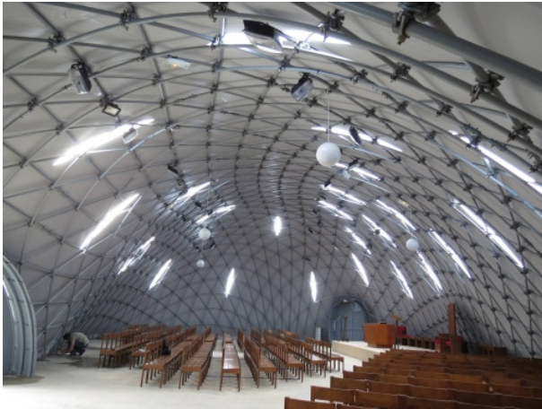
Figure 1: Ephemeral Cathedral of Créteil, France. This build is a first one of its kind, a grid shell structures made of composite materials [9]. It encompasses a surface area of 350 \text{ m}^2 .
