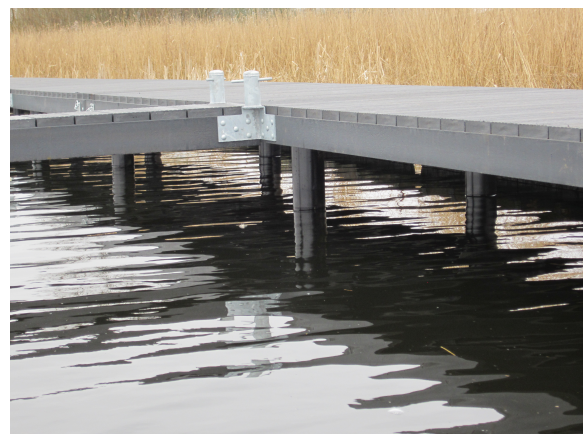
(b) View of a joint
