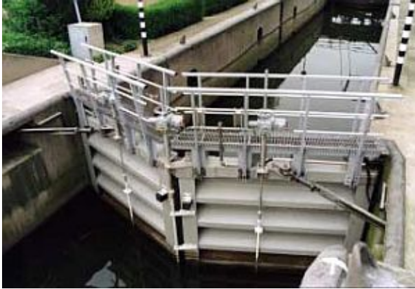
Figure 4: Spieringsluis, The Netherlands. This is the first FRP lock gate constructed and installed in The Netherlands. Two panels with a width of 3.5 m each compose the gate. The panels have a height of 6.5 m
