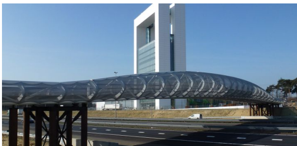
Figure 3: Floriade bridge, The Netherlands. This pedestrian and bicycle bridge can support vehicles up to 12 tonnes. It has a width of 6 m and spans 127.5 m. The GFRP deck rests on steel beams [10]
