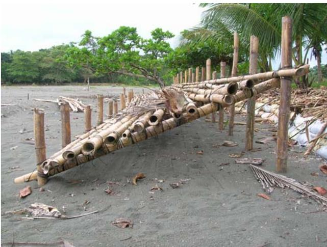
Figure 4.3: Timber revetment in front of the lodge
