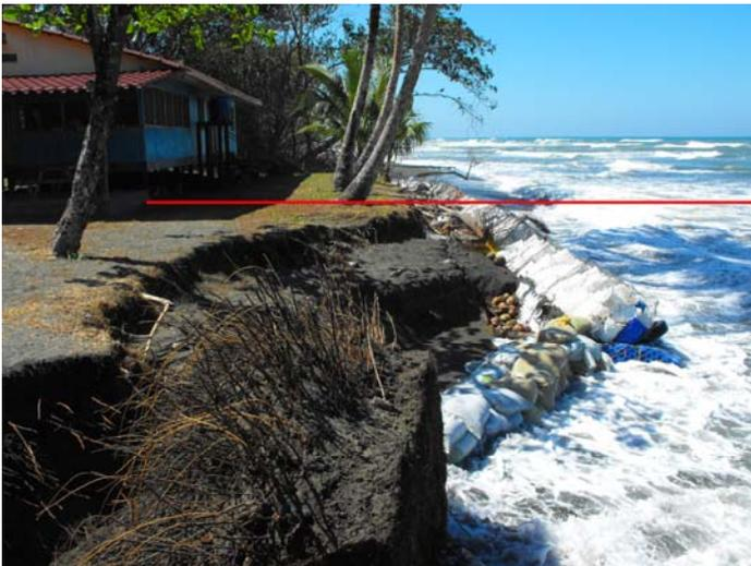
Figure 4.9: Coast profile (red line) examined in Unibest TC during a storm, protected with gibbons.
