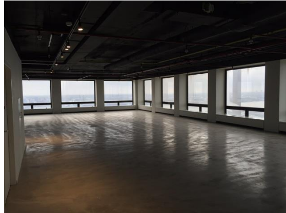
Figure 76 (right): Interior wideslab precast concrete floor spanning structural core and façade columns
