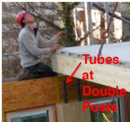
Figure 26: Placement of hybrid slabs on columns of façade elements (Tahan, 2012)
