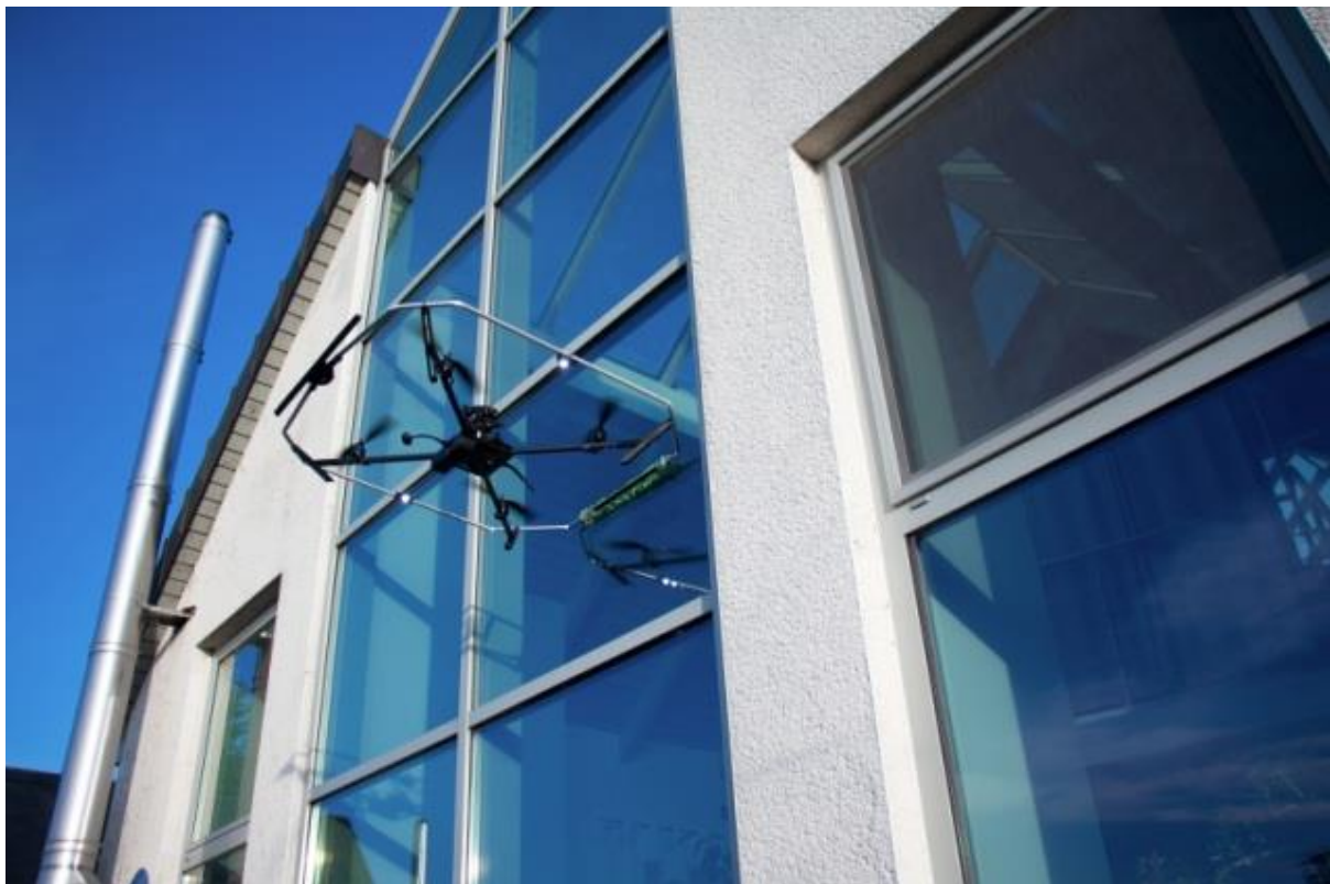
Figure 87: Window cleaning drone (Robinson, 2016).
