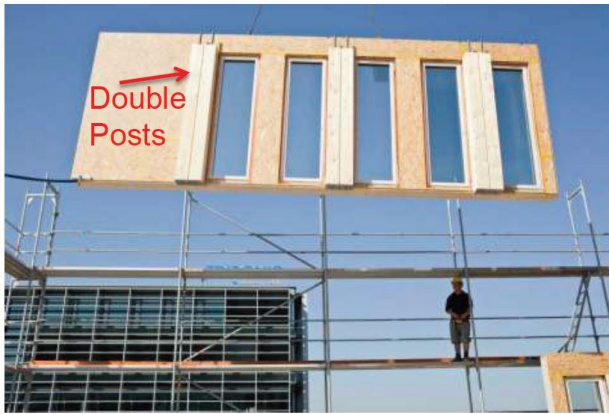
Figure 27: Façade element being lifted into place (left) (Tahan, 2012)
