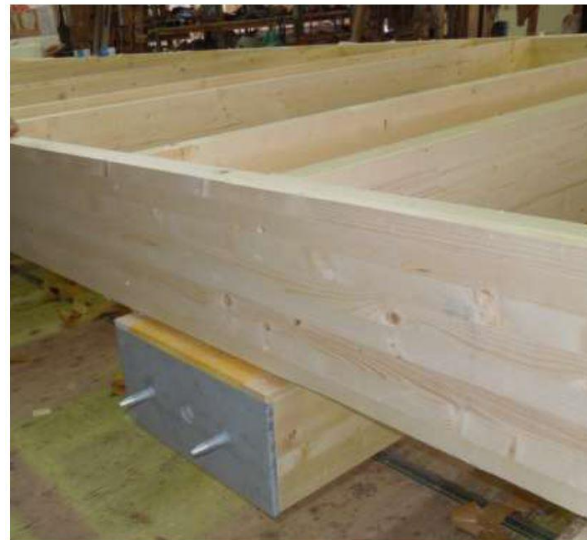
Figure 24: Hybrid slabs resting on wood double columns (left) (Cree GmbH, 2010)
