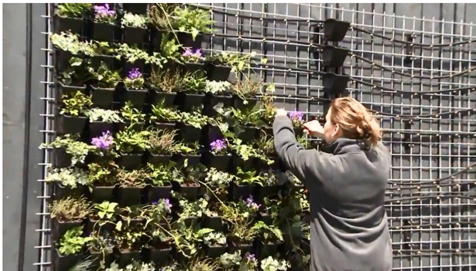
Figure 36 (left): The Bin Fen planter box system (O'Hara, 2012)
