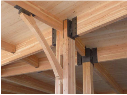
Figure 5 (left): Indirect connections (Evans, 2013)
