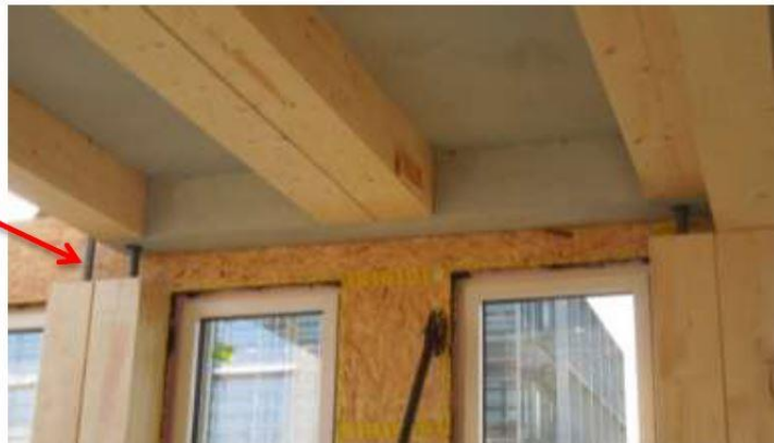
Figure 26: Placement of hybrid slabs on columns of façade elements (Tahan, 2012)
