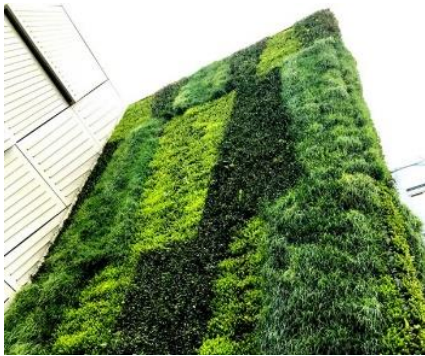
Figure 1.4: Living wall system gsky ProWallWater (Exterior Walls, n.d.).
