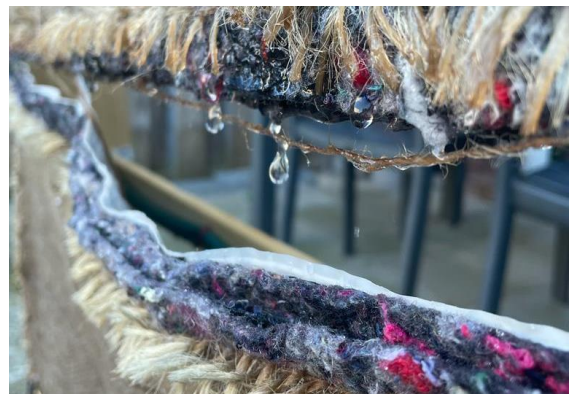
Water accumulation at the bottom of the mats
