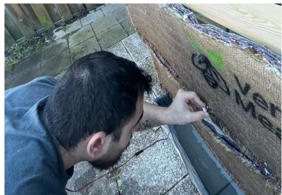
Preparing the moisture sensors
