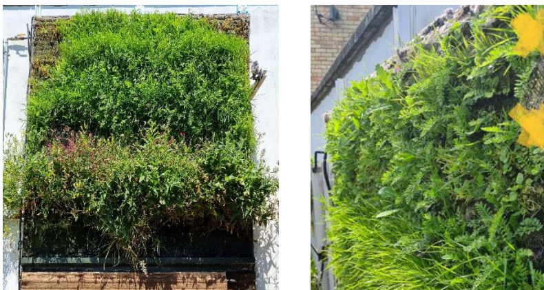
Figure 5.19: Living wall from London where the remote measurements took place (A. Law & R. Carlos, 2023)
