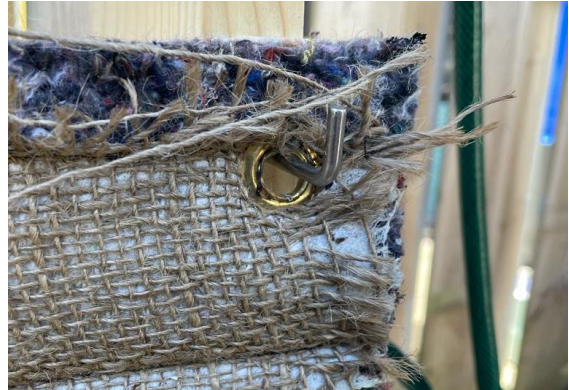
Connection of the mat to the wooden frame
