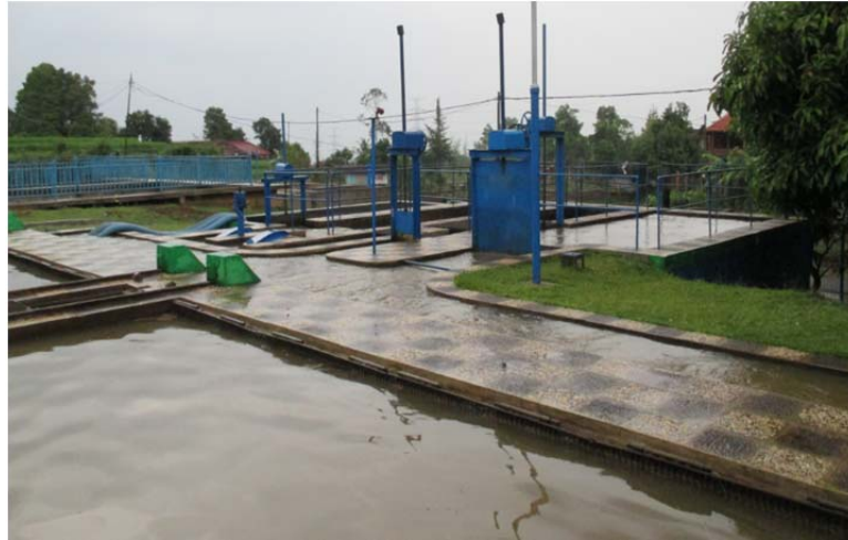
Figure 1. 14 Sluice Gates
