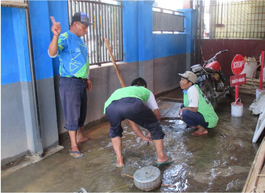
Figure 2. 12 Flooding caused by the air valve malfunction
