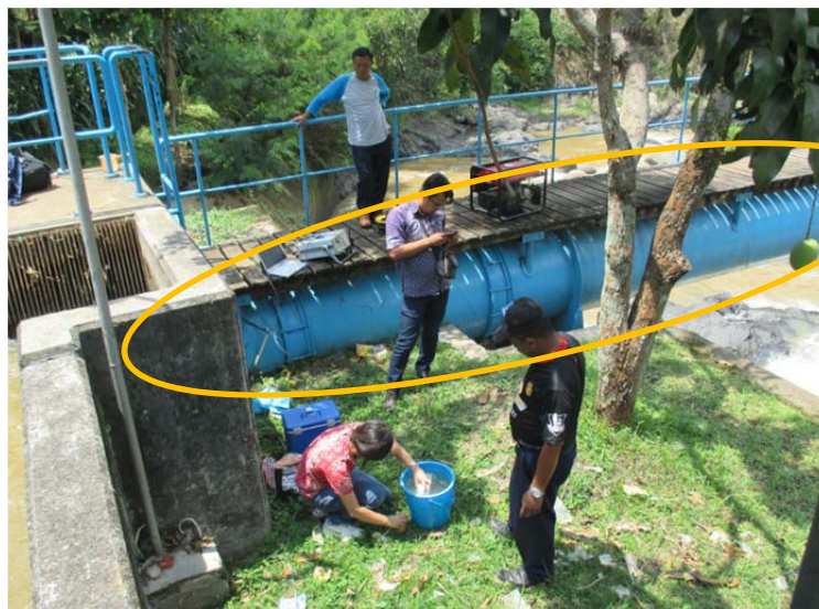
Figure 1. 9 Pipe Bridge
