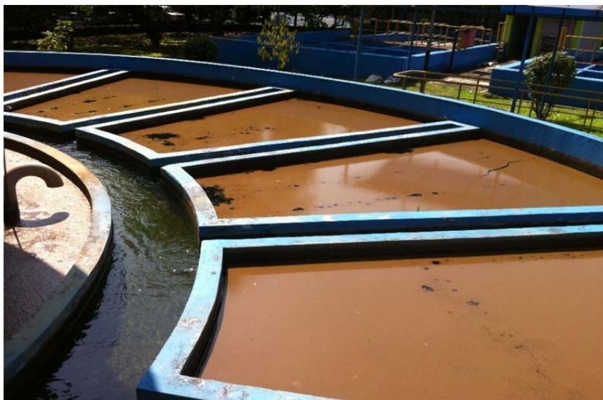
Figure 3. 23 Sludge layer on the top of the accelerators
