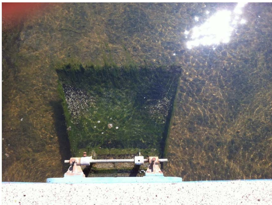
Figure 3.8 RSF 3 with algae growth
