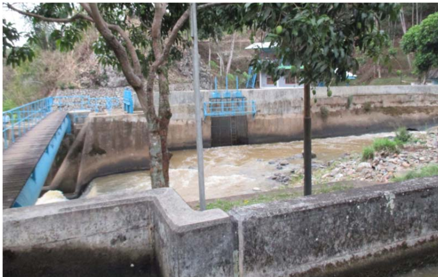
Figure 1. 7 Southern Raw Water Intake Structure
