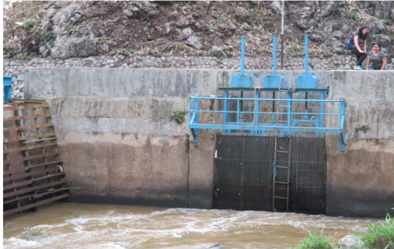
Figure 1.12 Intake Gate/Penstock
