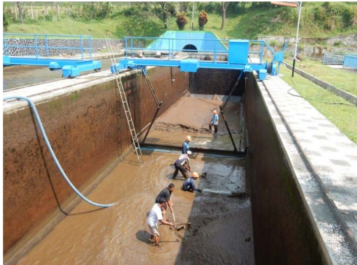
Figure 1. 19 Presedimentation Tank Cleaning Activity
