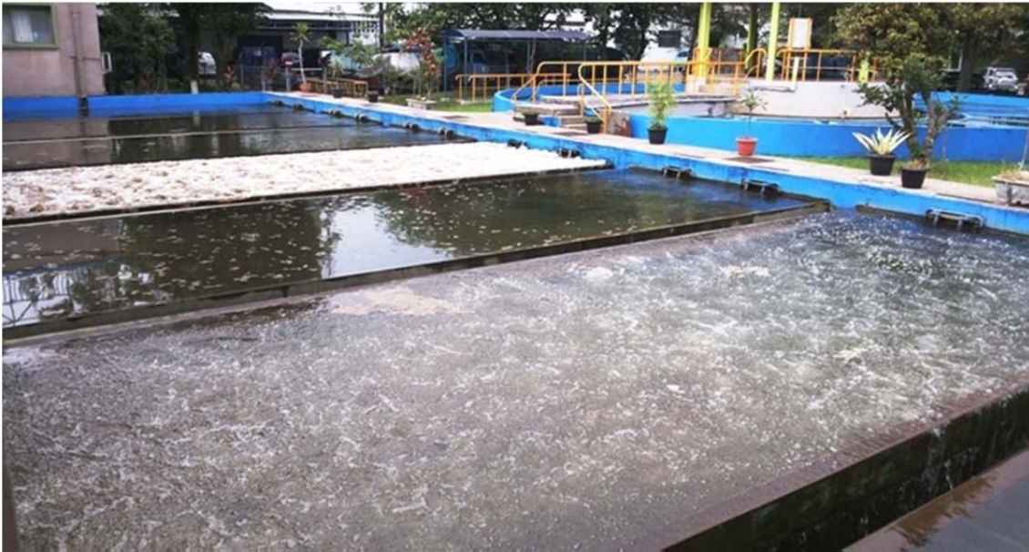
Figure 3.7 Backwashing of the filters.
