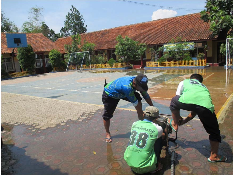
Figure 2. 11 Elementary school where the flood caused by the air valve malfunction occurred
