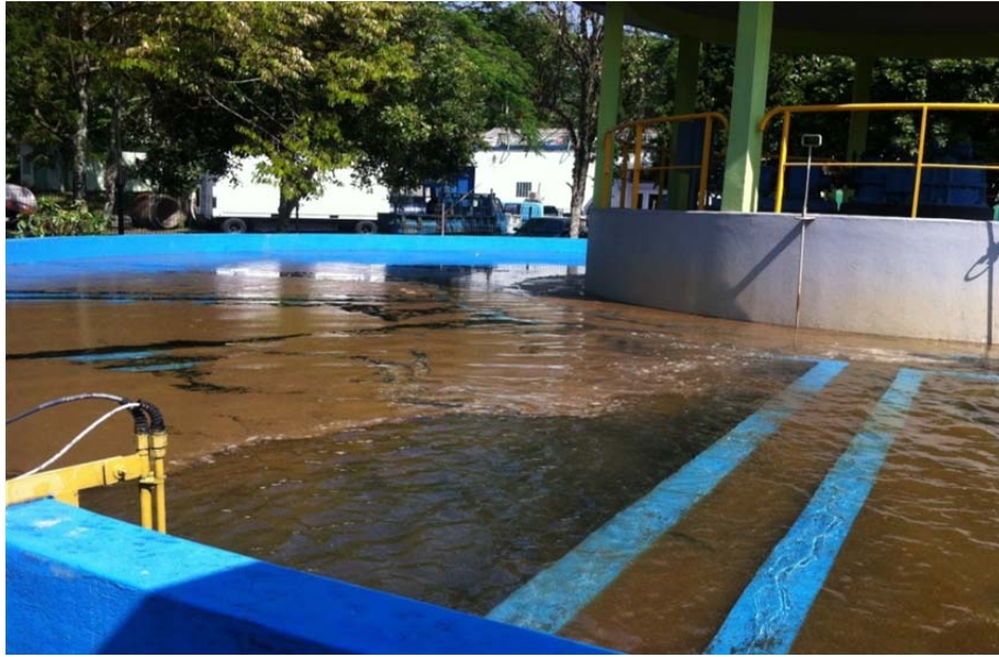
Figure 3. 27 Condition after cleaning
