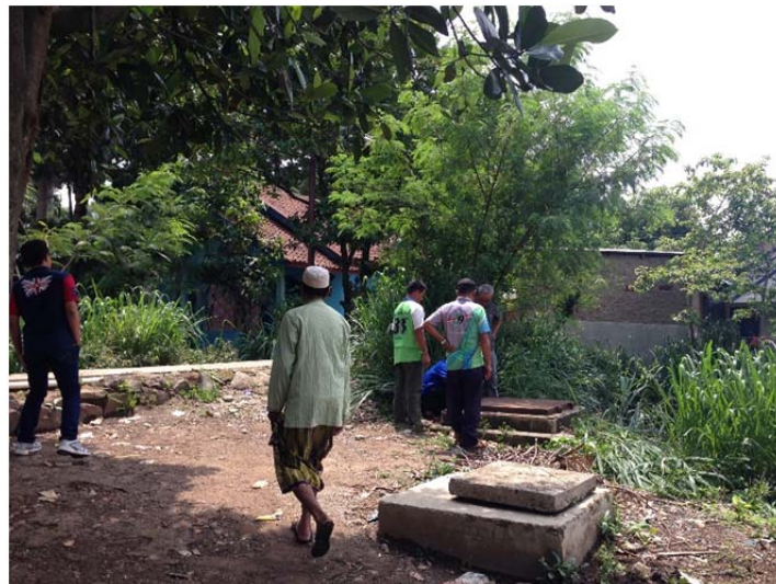
Figure 2. 15 Air valve in Kukje, located inside a village
