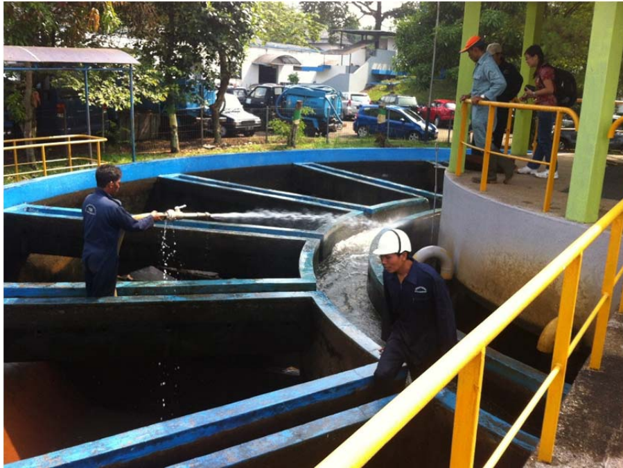
Figure 3. 6 Manual cleaning of accelator
