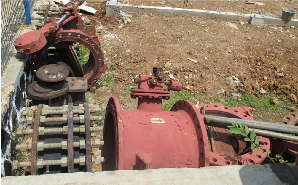
Figure 2. 6 Valves removed from pipeline stored in PDAM Cikalong
