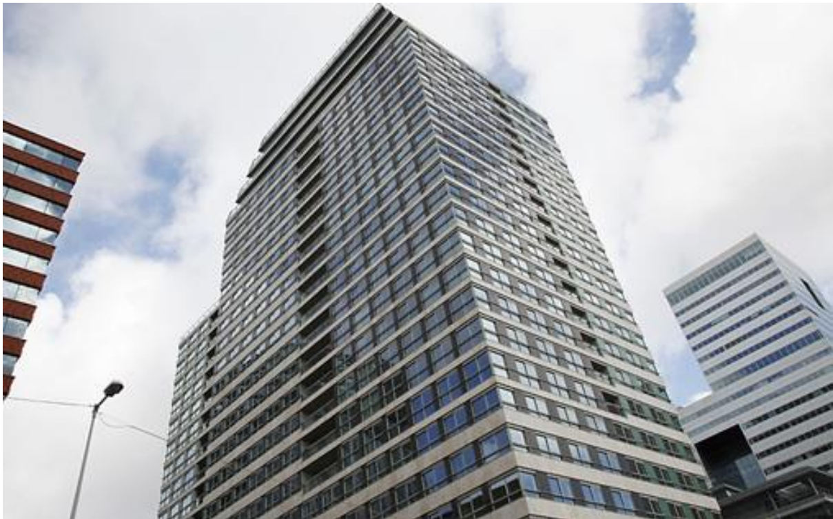
Fig 41. The New Amsterdam tower at the Zuidas
