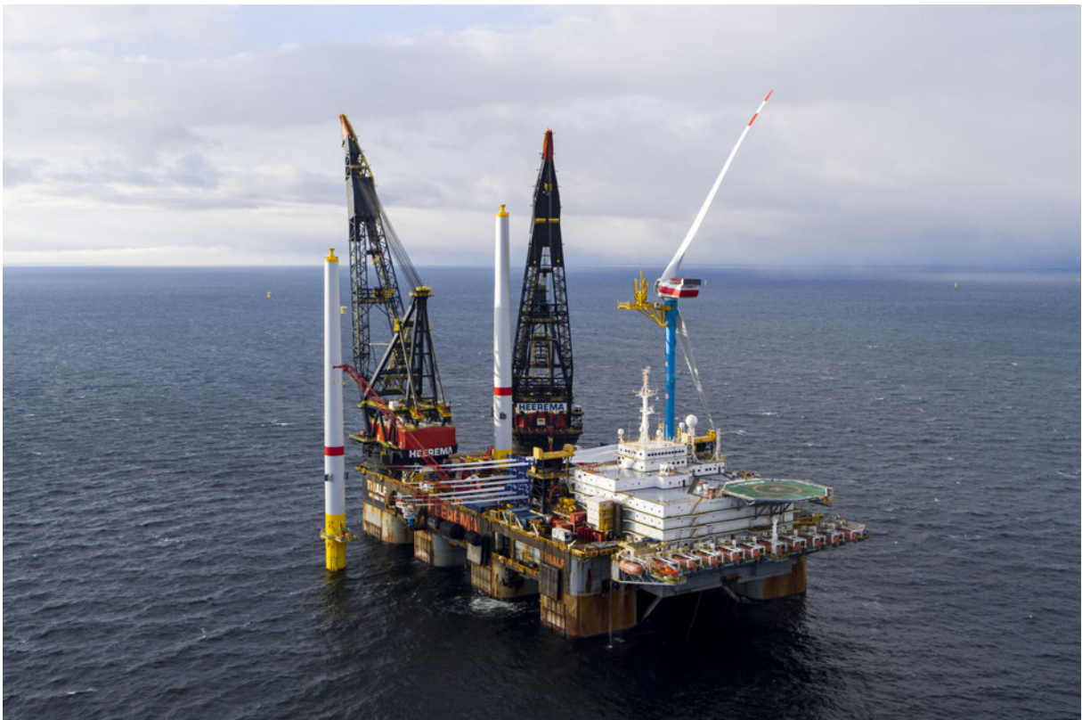
Figure 7.1: The Thialf performing an installation of a wind turbine generator
