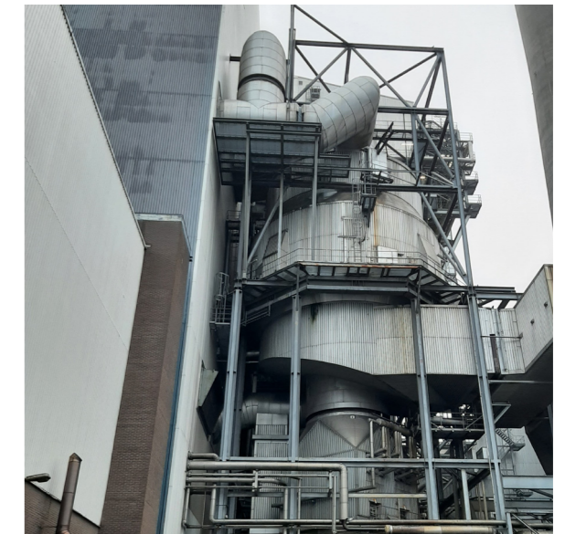
HEAT EXCHANGE AND TRANSPORT OF ASHES
