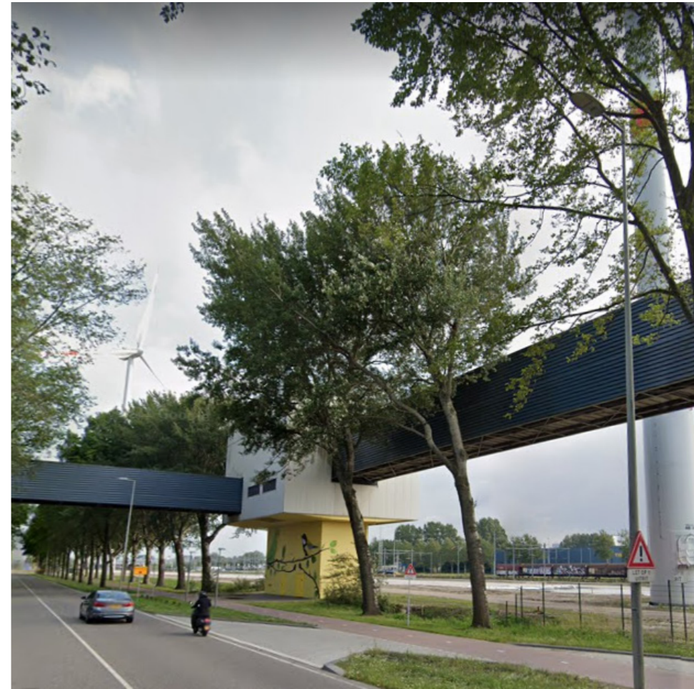
COAL CONVEYOR BELT
