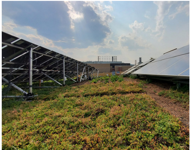
Figure 163: Extensive green roof with solar panels
