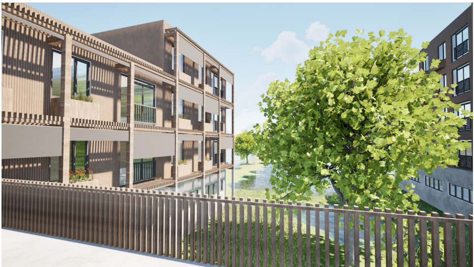
Figure 132: Shading structure on south facing façade
