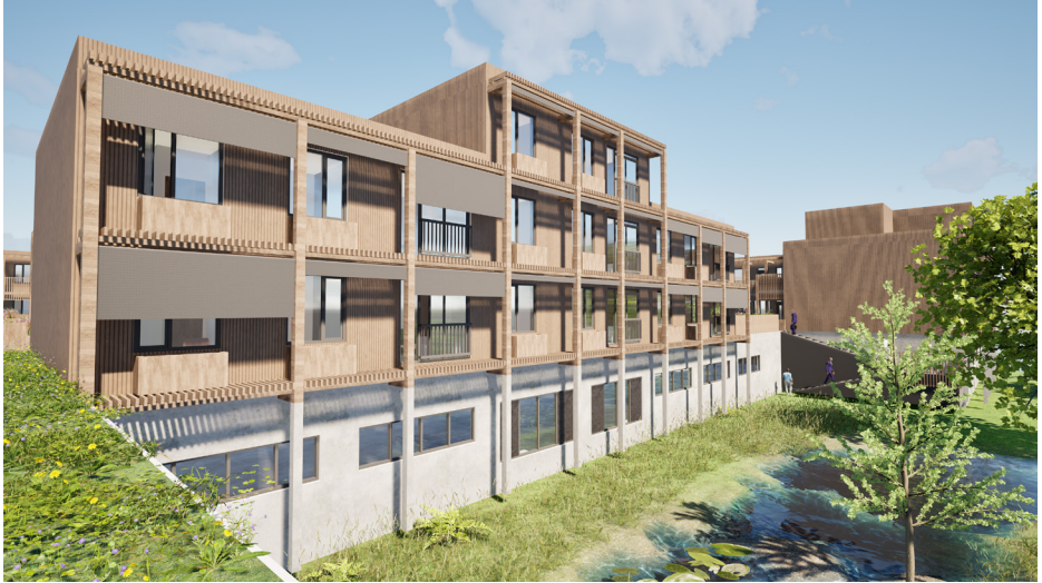
Figure 135: Building in dry state
