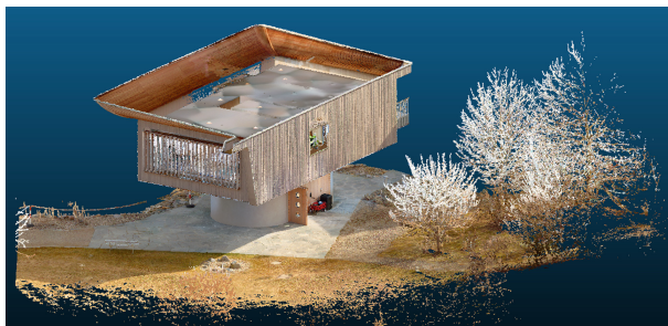
Fig. 1. The point cloud of the House “Haussicht”. It has 17 m long x7m width x 7m height, having 2 stories. The point cloud contains more than 7.5 million points.
