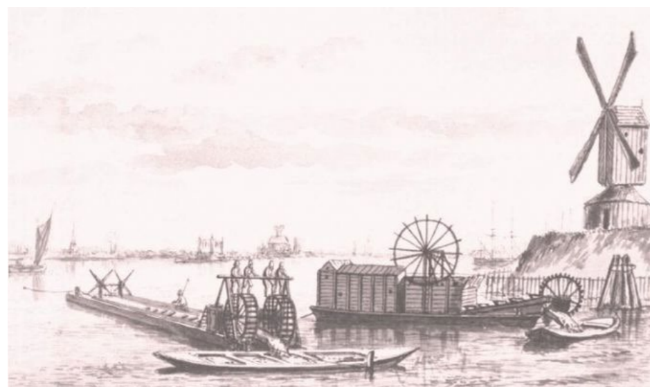
Figure 12. Mud mills keeping the Zuiderzee navigable for merchant ships (Source: www.hydro-international.com/content/article/the-hydrography-of-the-former-zuiderzee )
