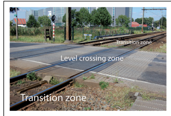
Figure 2. Level crossing with ERS (Harmelen LC, ProRail inspection photo).
