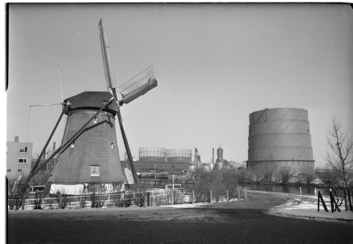
Municipal gas factory with spiral guided gasholder (1955) 24
