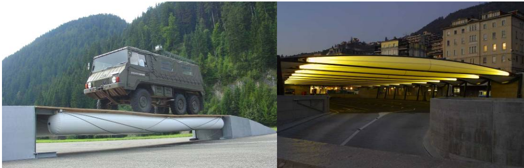
Figure 5. First applications of Tensairity in civil engineering: test bridge with 8 m span (left) and roof over a parking area in Montreux, Switzerland with 28 m span.
